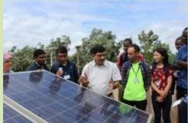
Roof-Top Solar PV System
